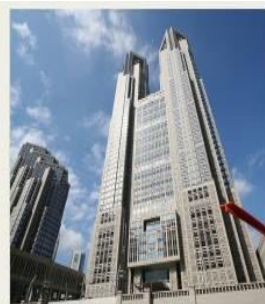
THE NEW TOKYO CITYHALL COMPLEX | TOKYO, JAPAN
